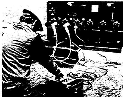
Figure 26. Testing a Cable.
